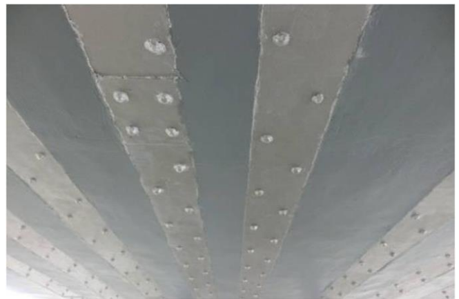
Fig. 27. Steel plate strengthening at the soffit.
