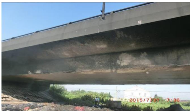
Fig. 6. Fire-damaged span 1.
