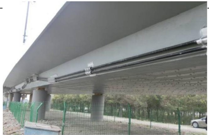
Fig. 26. External prestressing strengthening at webs.
