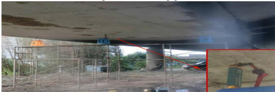
Fig. 16. Installation of the deflection gauges.
