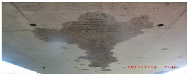
Fig. 7. Fire-damaged span 2.
