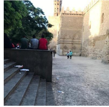
Figure 28. Dirty Pavement & Garbage
