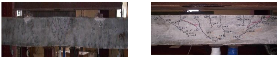
Figure 10. Flexural failure: Crack pattern at failure for B6
