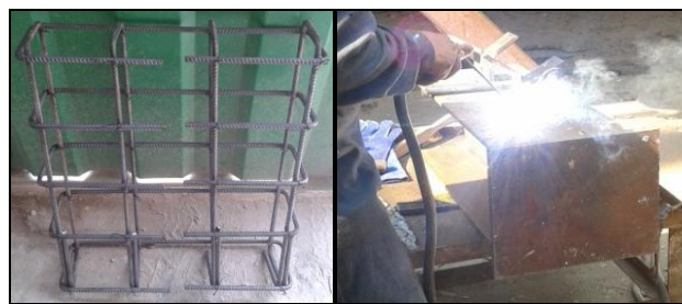
(a) Assembling the RFT (b) Welding the
