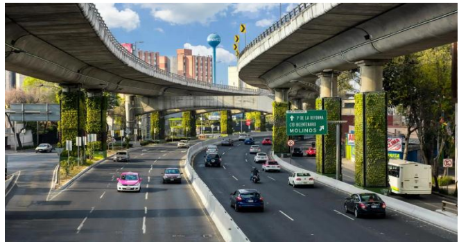
Figure 19. d) A busy highway in Mexico City has 1,000 pillars covered with vertical gardens and below bridges planting [26]
