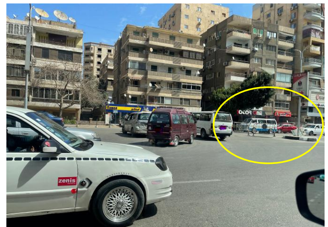
Figure 33. Using movable metal fences to allow safe U-turning to El-Nahas Street from El-Tyran extension Street since the median design, and dimension are not adequate [17] (9/3/2023).
