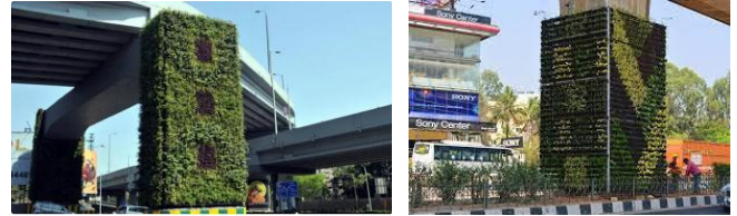
Figure 19. b) A vertical garden on the pillars at a bridge close to COEP in Pune, India [24], c) Bangalore, India, gets its first vertical garden on flyover pillars in an attempt to reduce pollution [25]
