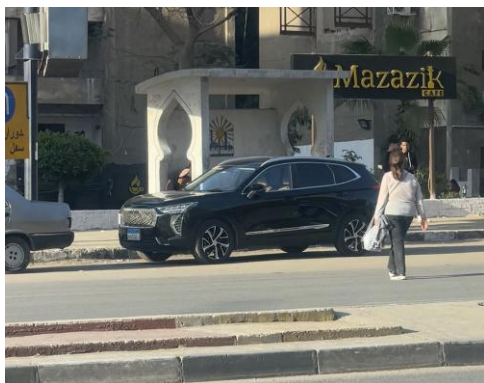
Figure 36. A bus stop is currently found in part of the street from the third development stage [17] (9/3/2023).
