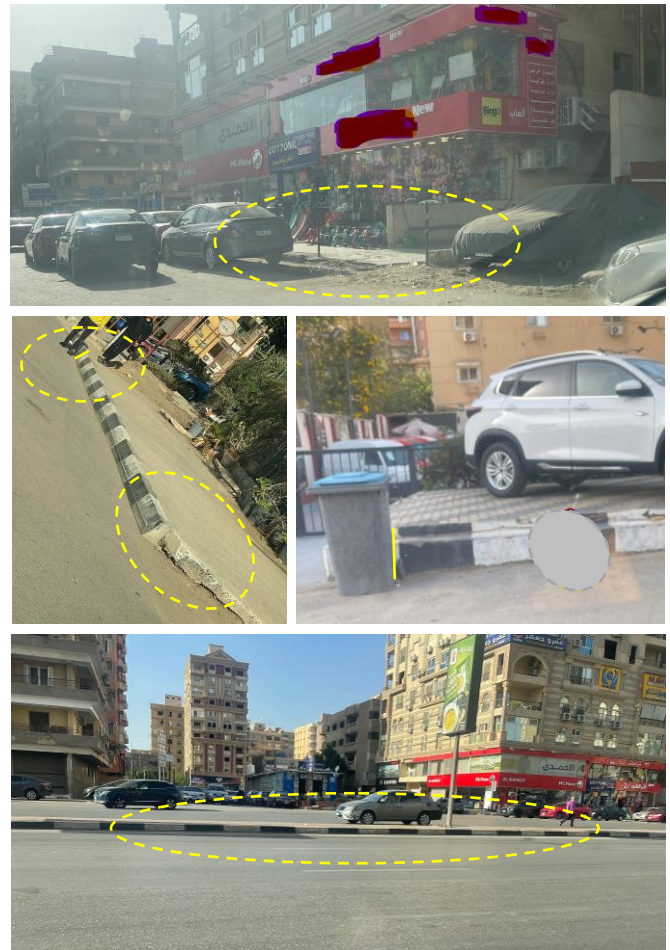
Figure 34. a), b), c), & d) Sidewalks and curbs various photos showing their current state, height, finishes, and unauthorized occupations marked using yellow shapes [17] (26/4/2023).
