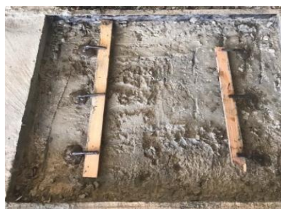
(c) Install the dowels by epoxy
