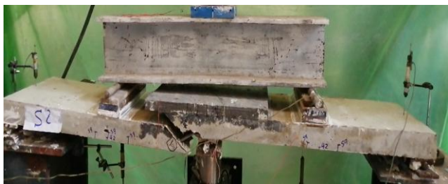
(b) Crack pattern of specimen S_2
