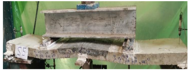
(e) Crack pattern of specimen S_5
