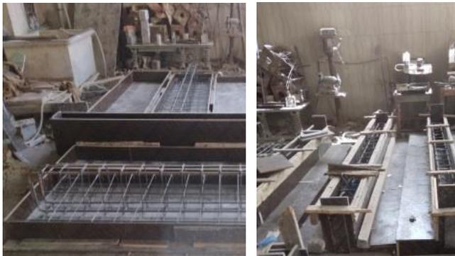
(a) Installation of reinforcing mesh inside the formwork (b) a final view before casting concrete
