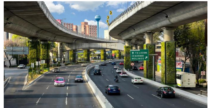
Figure 19. d) A busy highway in Mexico City has 1,000 pillars covered with vertical gardens and below bridges planting [26]
