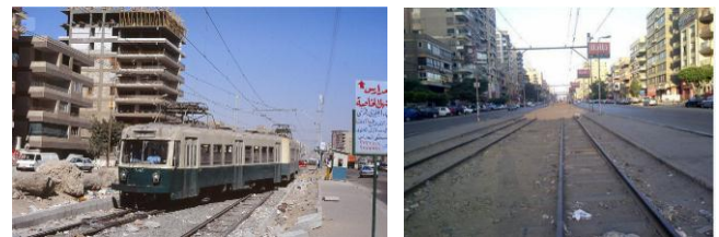
Figure 2. a) & b) The axis with a metro in its middle [12] & [13].
