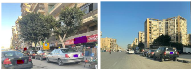
Figure 22. a) & b) Some parts of the street sidewalks with the landscape, however, it is not enough to give the street the required visual and environmental effect [17] (9/3/2023).
