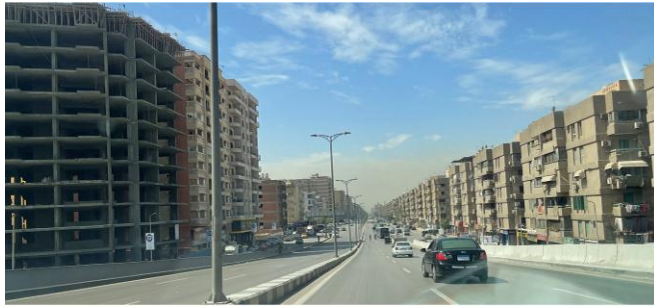
Figure 4. a), b), & c) Sectors on Mostafa El-Nahas axis showing the bridges [16] & [17] (12/2/2023).
