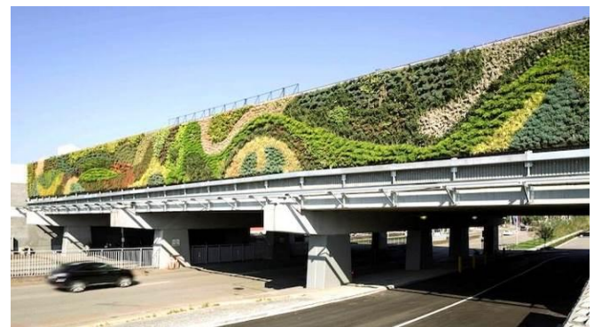
Figure 19. e) The biggest green wall in North America was finished in Vancouver, in Surrey British Columbia. It is a double-sided, 10,150 square-foot green wall made up of 50,000 individual plants, the majority of which are indigenous to British Columbia [27]
