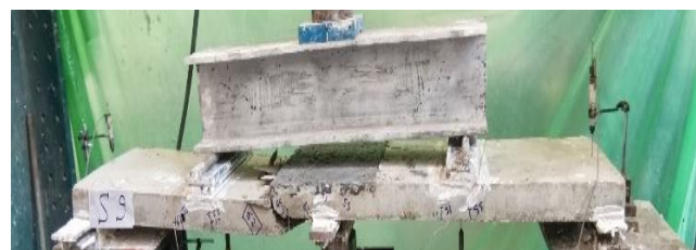
(j) Crack pattern of specimen S_9
