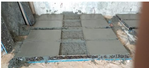
(a) Finishing the surface and roughing the strengthened area
