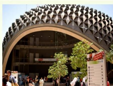
The use of a dome with a projection to provide shade and reduce the heat inside
