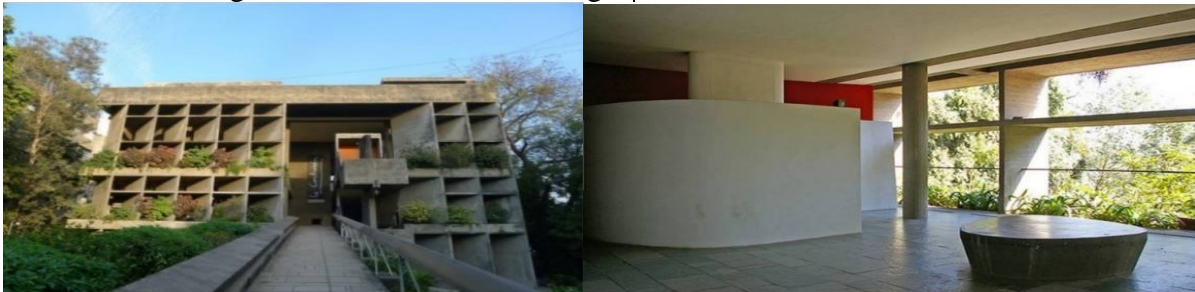
Photo No. (4) of " The Mill Owners' Building " for Le Corbusier, in which the distribution of interior designs is described as a play of volumes in light and shade, and this building is a good example to reduce energy consumption and maintain natural ventilation, Source: https://www.archdaily.com/464142/ad-classics-mill-owners-association-building-le-corbusier
