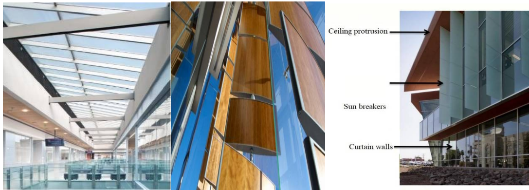
Photo No. (6) illustrates the use of wood as a natural non-toxic and non-radioactive material for chemicals in the occasional wooden blinds used to shade the facades of the University of Arizona building, Source: architizer.com/projects/university-of-arizona
