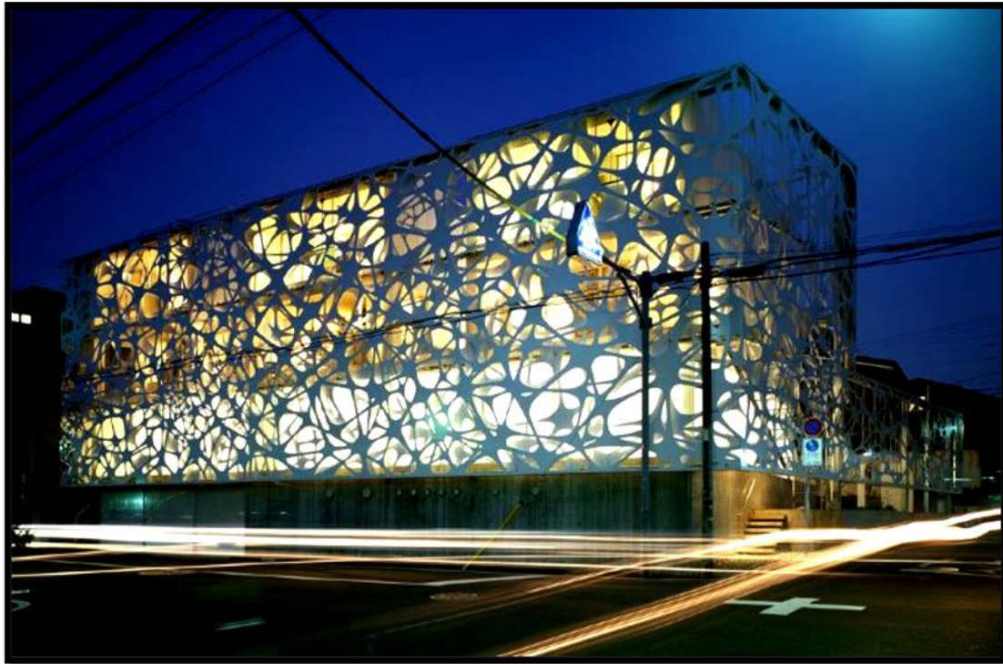
Fig.(6b ) Project AIRSPACE TOKYO was designed by FAULDERS STUDIO. He created a digital design for the intertwining Voronoi pattern representing plant biocytes. Night lighting passing through the Voronoi holes creates a mysterious feeling of movement. On the left is a schematic diagram of the Voronoi diagram and the bottom of the cube building inspired by the Voronoi. Ryota Atarashi(2012)Thomas Faulders Architecture retrived from arch2o.com on 9/1/2021
