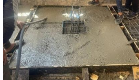
(b) Casting of normal strength concrete
