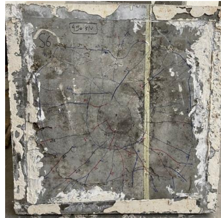
(f) Crack patterns of S6
