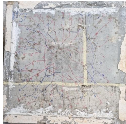
(g) Crack patterns of S7
