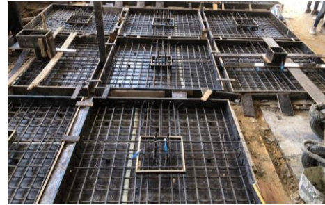
(a) Installation of reinforcing meshes inside the formwork and mold
