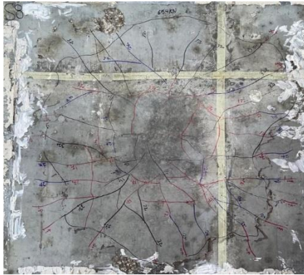
(h) Crack patterns of S8
